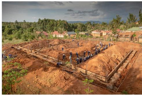
These photos show just how complex the earthworks have been. An enormous amount of soil has been moved to dig the deep excavations for the foundations.
